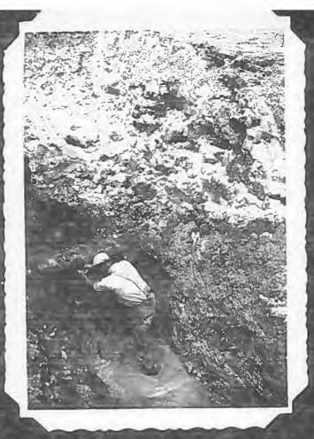
8-inch waterline connection and sewer junction at upper end of "Center St.:"
