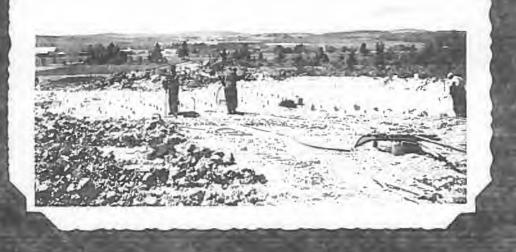
Laying 24-inch sewer on "Centre Street"Rock subgrade for street in foreground.
